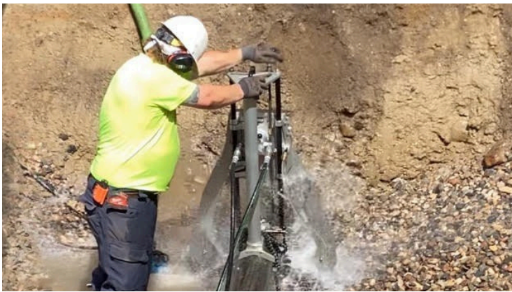
ALP's new diamond wire guillotine saw is improving safety and efficiency.
